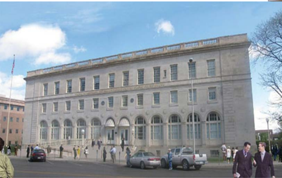
The Wayne N. Aspinall Federal Building and U.S. Courthouse in Grand Junction, CO, which GSA is aiming to turn into a Net-Zero Energy usage historic building. (Photo courtesy of GSA)
